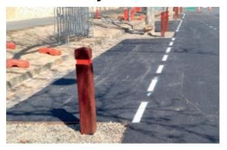
High profile renewal of bluestone kerb and water table infrastructure project, with minor ancillary works between Wellington Square and Montefiore Hill. Scope includes road resurfacing, line marking, and heritage kerb 'bluestone' works, while navigating major tree roots and underground services.
