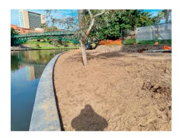
The project is new and upgrade work and will deliver a structure (piled retention system) to stabilise and prevent further slumping of the riverbank and pathway near the University foot Bridge.
